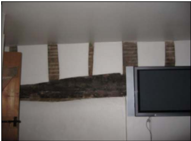
East wall with tie beam, which retains some smoke blackening.
