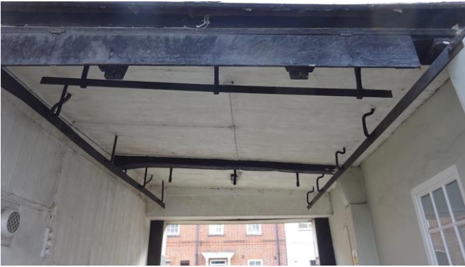
Trackway with iron hooks, used by the butcher to move carcasses.
