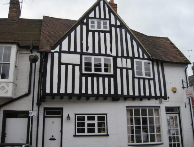
14 and 14a Friday St – an elegant Tudor house, with moulded jetty beams.
