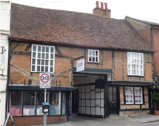
Old Broad Gates, Market Place. The 1353 jettied wing is on the left of the passageway. What remains of a crown post roof has been mutilated by the large Georgian window. One gothic arch door still leads into the ground floor room; a second one is blocked.
