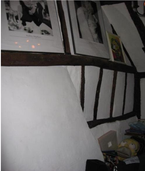
The rear bedroom has a traditionally framed gable wall, although of lighter scantling, with the stack from the ground floor rising against it and then disappearing behind the tie beam to the outside of the gable wall.
