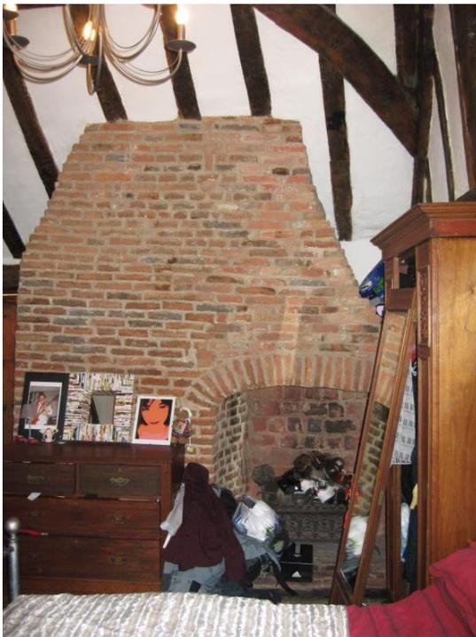
The front bedroom has a substantial, 2" 'Tudor brick' fire place with a hearth and flue to one side, which allows plenty of space for the main flue from the ground floor fire place to be accommodated.
