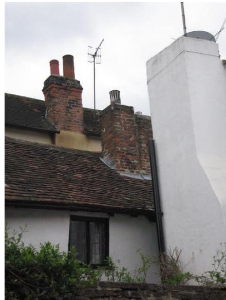
**East, front elevation of No. 60, its brick stack adjoins that of 58, just visible behind the white rendered rear stack of No 78; The central stack on the tall roof behind is that of the adjoining 'Rose & Crown' PH**
