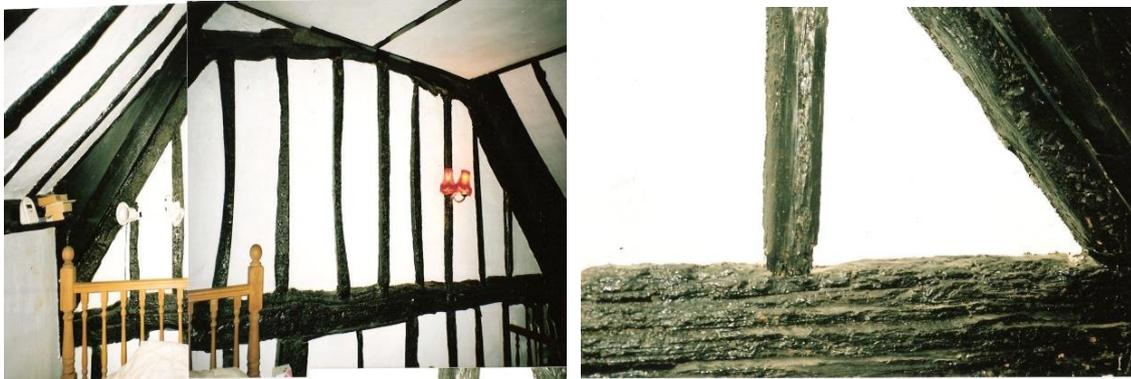
South facing gable of No. 64, seen from inside No. 66. NB the heavily weathered timbers
