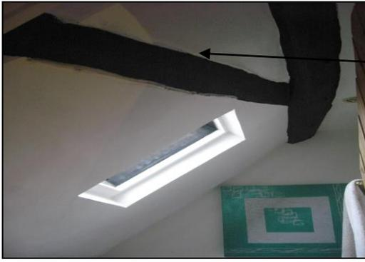
First floor: rear/north part of the roof (visible only in the bathroom) with a substantial purlin and straight wind brace in the roof slope. The pegs, visible in the underside of the purlin, for holding the common rafters, are widely spaced and are strong indicators of a formerly thatched roof.
