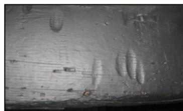
**Left:** Soffit of transverse beam with empty mortise where the wall timber post was removed. There are also a number of smaller mortise slots of former wall studs.
