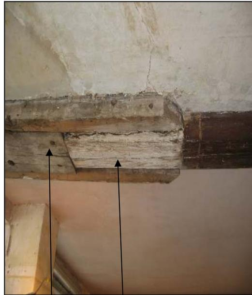
F. floor, front room ceiling beam is 10" wide and shows where the former north wall was located underneath it (lime mortar of former 22" brick wall) when the front was rebuilt further north out onto the 'lord's waste', ie. the present pavement.
