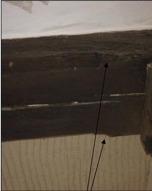
G. floor, front room ceiling beam is 1 foot wide and has chamfers with step & run-out stops at both ends. These are known from the 14<sup>th</sup> to 17<sup>th</sup> C. ( see Linda Hall 'Period House, Fixtures and Fittings' P 159 )
