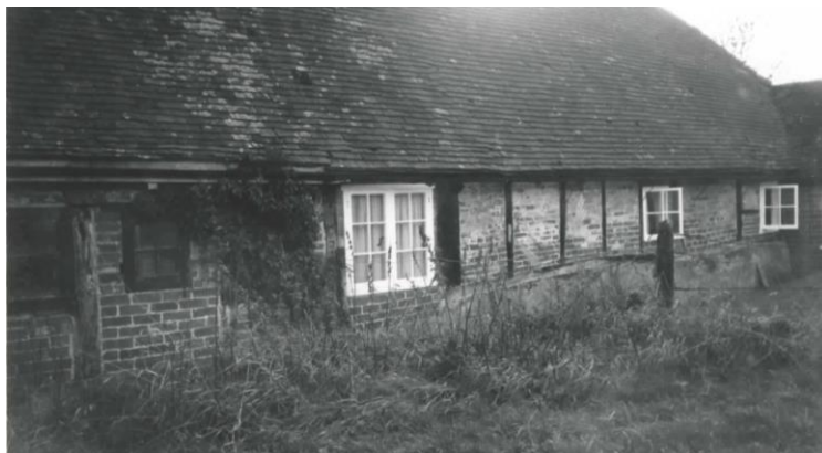
Back view of Hunt's Farmhouse, note the low eaves
