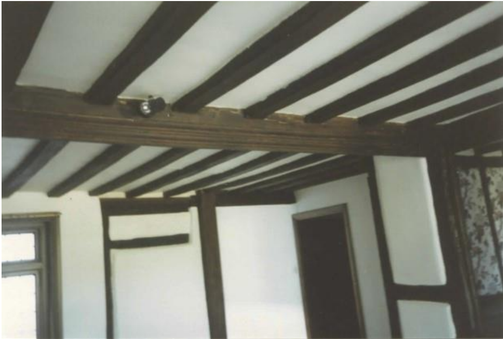
Roll-moulded spine beam in the hall
