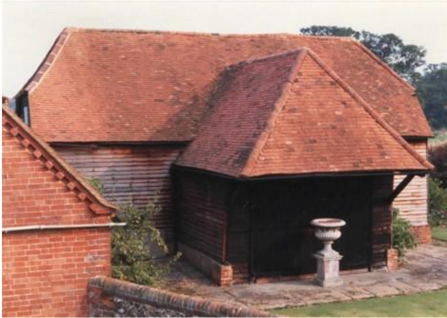
Barn, west side with large porch
