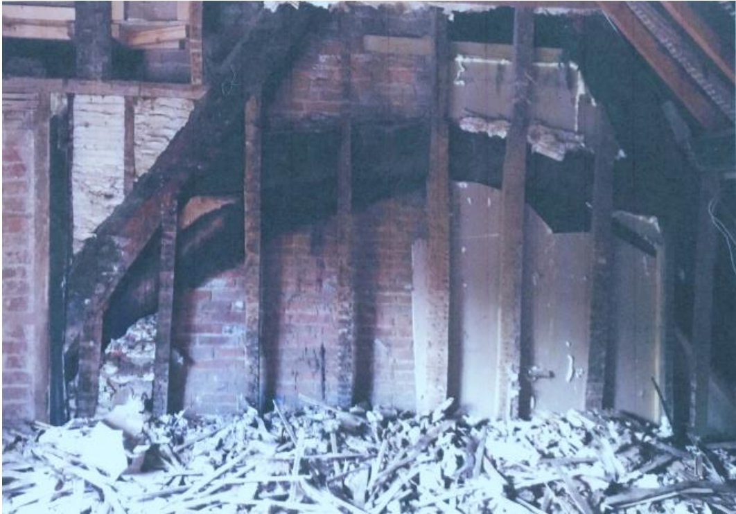
Hunt's Farmhouse – Eastern Truss discovered during works in 2020 by new owners
