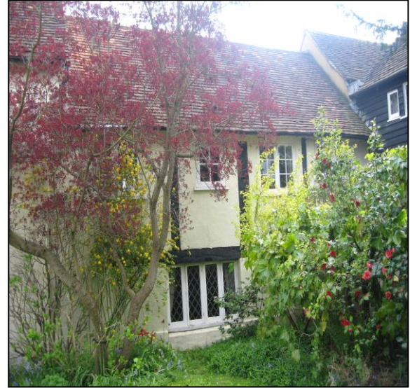
Rear/west elevation of the 2 medieval bays
