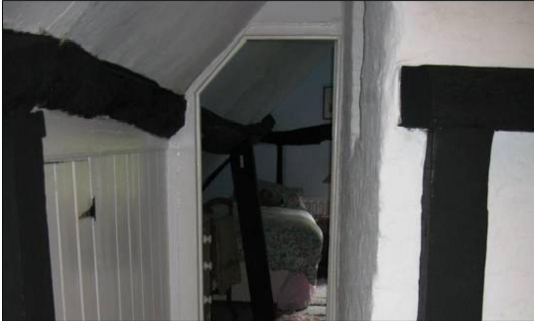
**Attic showing cut collar in front of the stack on the right, supported by a queen strut, bowing purlin on the left with modern supporting strut in the south bedroom beyond the stack**
