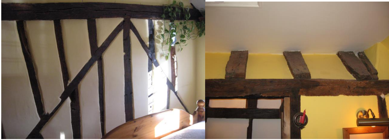
No 60, left: First floor, front bedroom. Stud wall between Nos. 58 and 60 West Street Right: First floor, view of roof rafter of front range resting on the wall plate, seen from the back bedroom.
