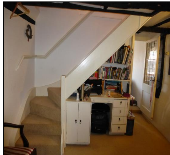
Rear room; stairs built against the stack
