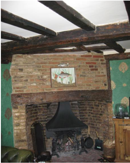
No. 60: Corner brick fire place in G.F. Axial ceiling beam with chamfer and stop
