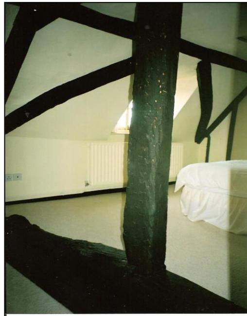
The c. 7 feet tall crown strut posts are the central part of the trusses, which form the bay divisions of the timber framed house; here seen in the attics. The l.h. side, painted white, in No. 28; the r.h. side, painted black in No. 29.
