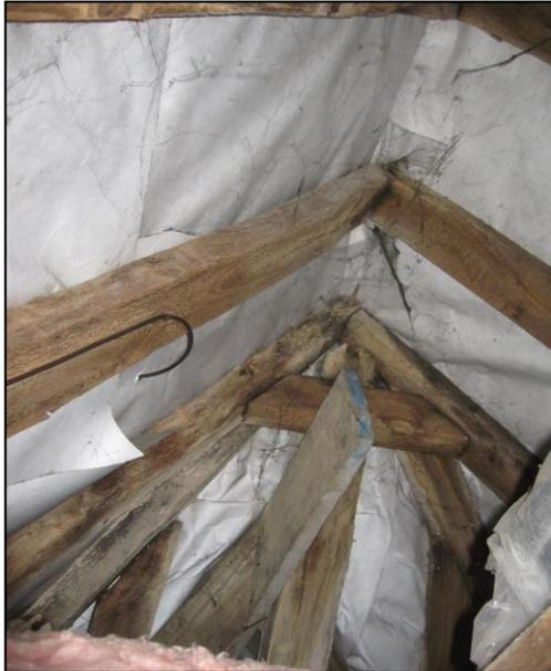
Pegged rafter roof above Bay I, looking south towards hipped end. There is a saddle between the last pair of rafters to support the hip rafter. (Ignore the board below the saddle, not part of the original roof structure)
