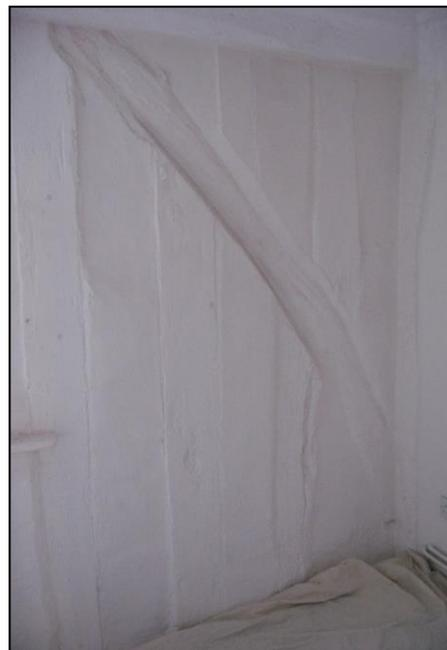
South end gable wall of Bay 1 with blocked window, studs and long wall brace, seen from first floor room of the adjoining 19<sup>th</sup> cent. building.
