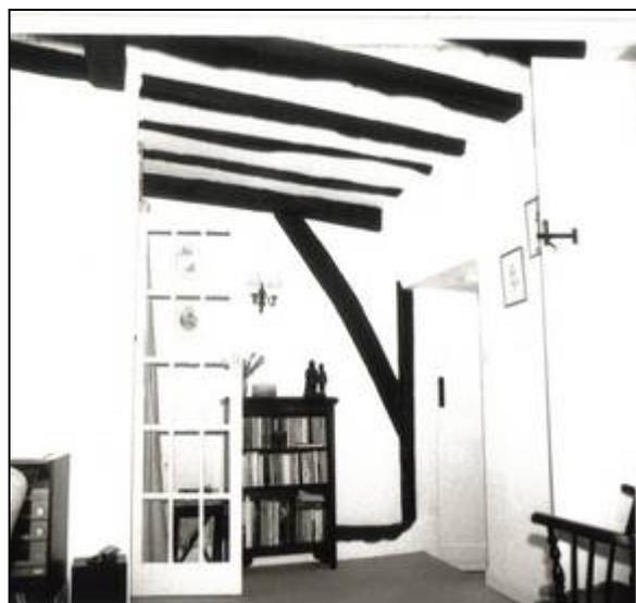
Interior of No. 17. The long arch brace in the side wall is typical of a medieval timber frame. Two other examples in Henley date from 1438
