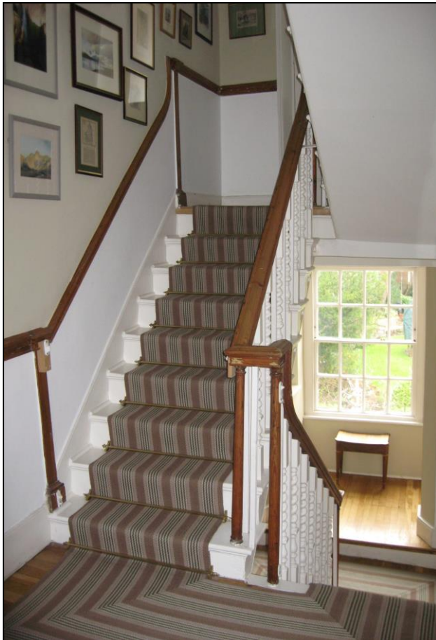
Stair case at first floor landing; details of two types of balusters (right above); toad-back hand rail ramped over newel post halved into the stair wall (right below)
