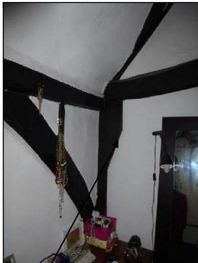
First floor room: wall post with wide jowl to support both plate and tie beams. Also note large, curved wall brace. The weathered post and brace below are the original east wall of No. 63 but are now only visible in the bedroom of No. 65.
