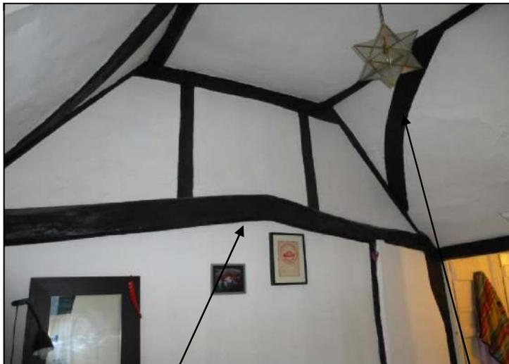
The cambered tie beam supports the queen struts of the clasped purlin truss. Also note the wide, curved wind braces. All timbers indicate a well built, substantial structure, probably of mid-15<sup>th</sup> date, now occupied by the mid 19<sup>th</sup> C brick terrace at 57/59/61. The latter are still bounded by the Parsonage Way on the west, the side entrance to the former large Rectory grounds.
