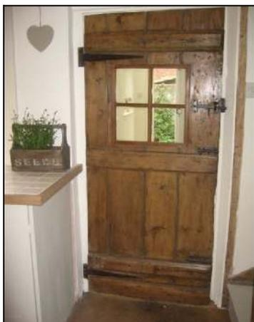
Ledge and plank kitchen door with long, round ended strap hinges, probably machine-made replacements. These were in use throughout the 18<sup>th</sup> and much of the 19<sup>th</sup> centuries.
