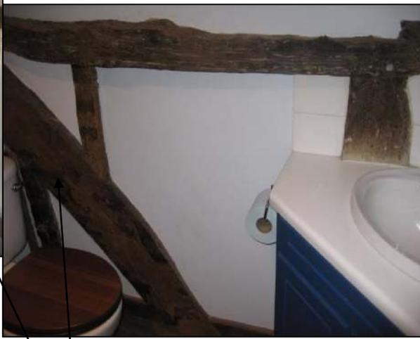
Long arch brace seen in two parts on the stair landing and in the rear bathroom.
