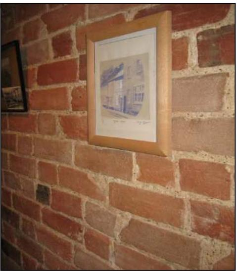
Ground floor east wall. These large bricks, mainly laid in an irregular Flemish bond, indicate a late 18<sup>th</sup>/early 19<sup>th</sup> C date for this wall, which was erected below the sooted tie beam, once the centre of the medieval hall.
