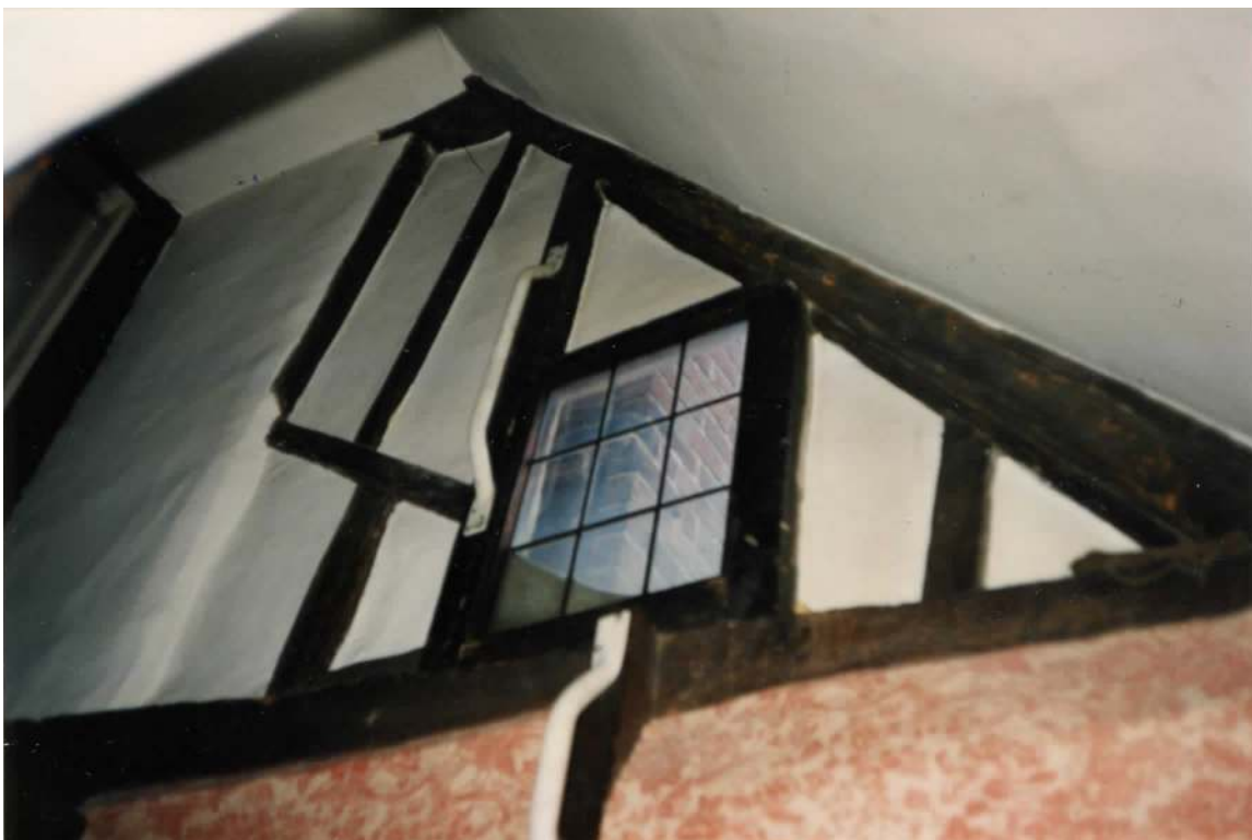
Part of the roof truss, looking west
