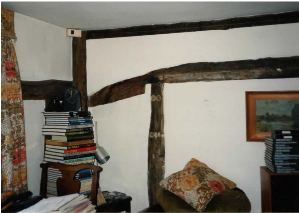
No 23 Friday Street - Ground floor, back extension, east wall
