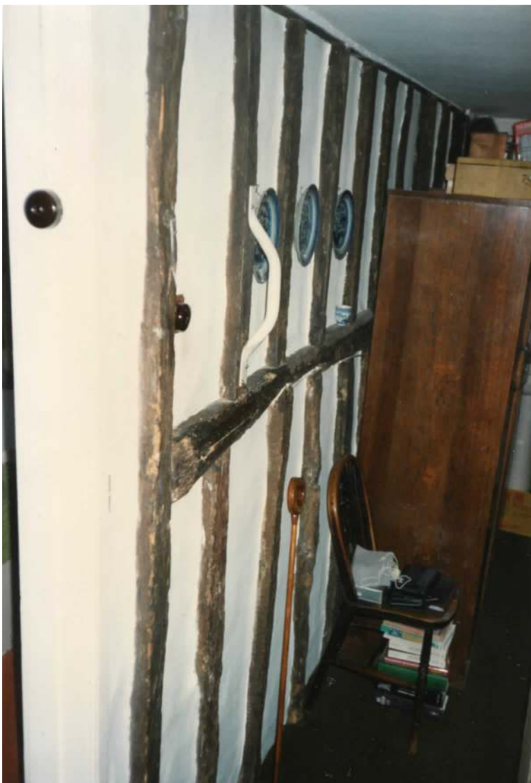
First floor, back extension, internal partition
