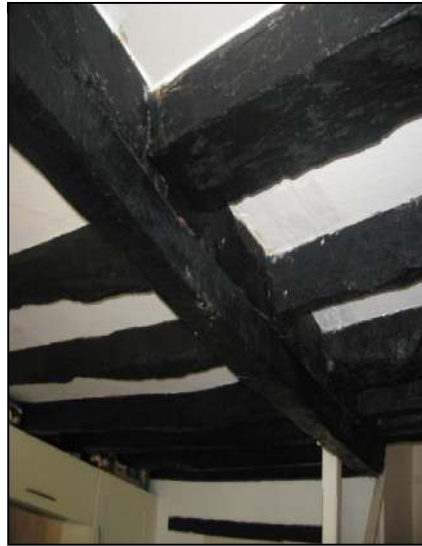
and central axial beam with uneven joists
