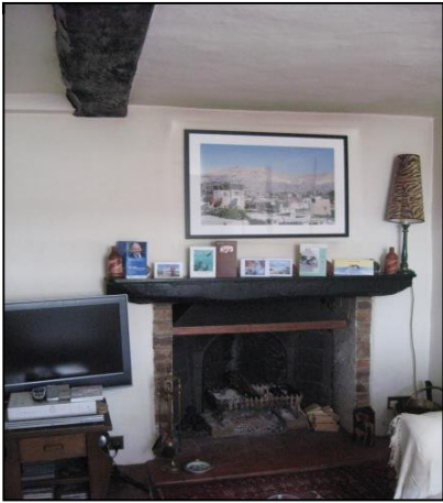
Ground floor front room, north wall with 1.06 m wide and 0.58 m deep FP East wall with three narrow studs
