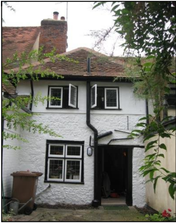
Hipped C.18 th kitchen extension. Note 3-flue stack View of the front roof, looking east towards No. 23/25 - with gap visible behind the collar
