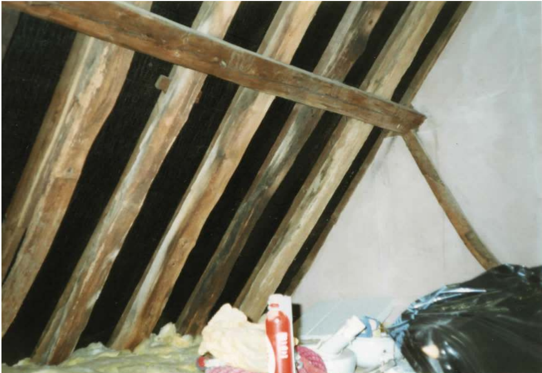
Above: Looking into the Apex of the Roof of No. 19
