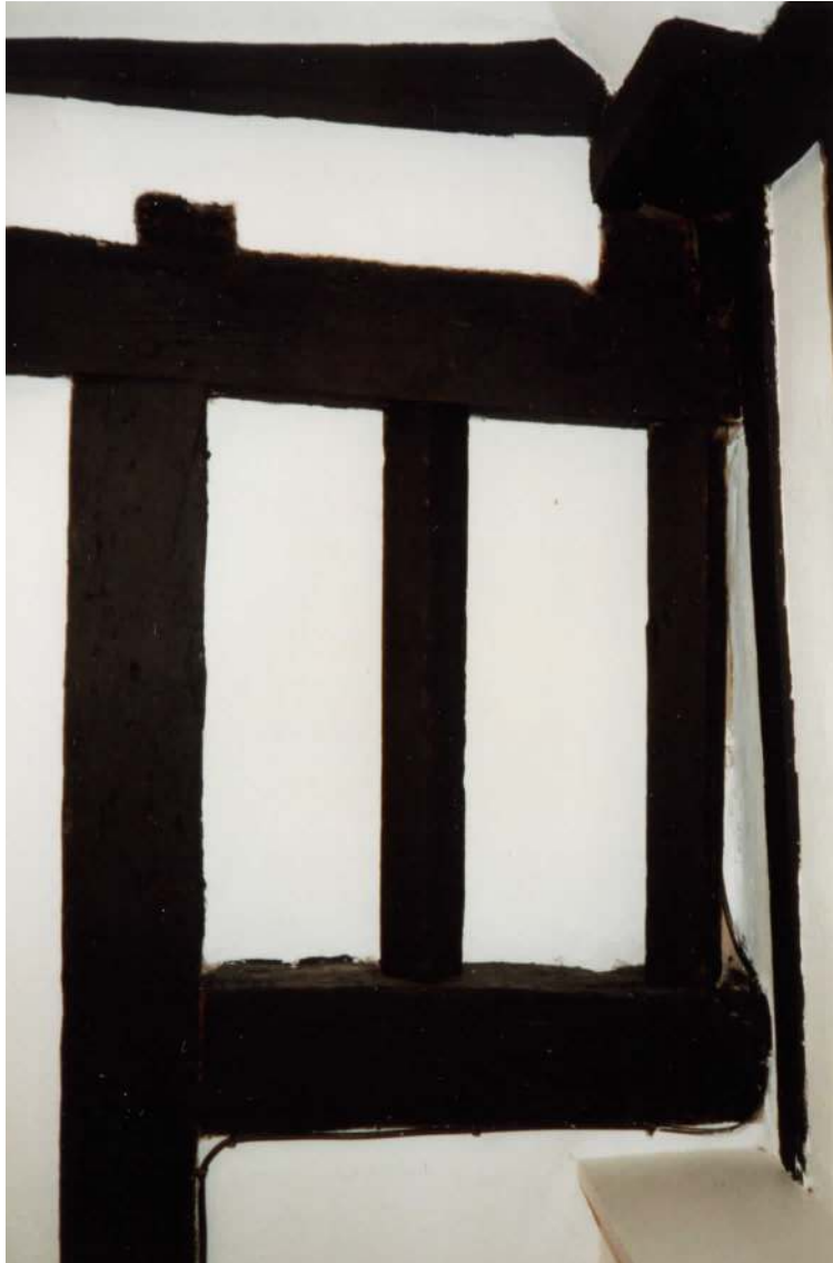
Half of Mullion Window in West Wall of No. 19. This Window belongs to No. 17 and was Partially Blocked when the Back Bedroom of No. 19 was built over the Kitchen. The other half still serves as a Window in the Rear Wing of No. 17
