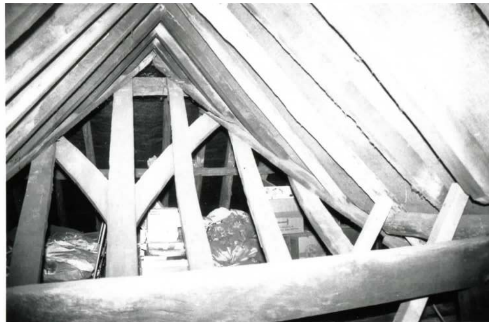
View of Central Truss from back wing
