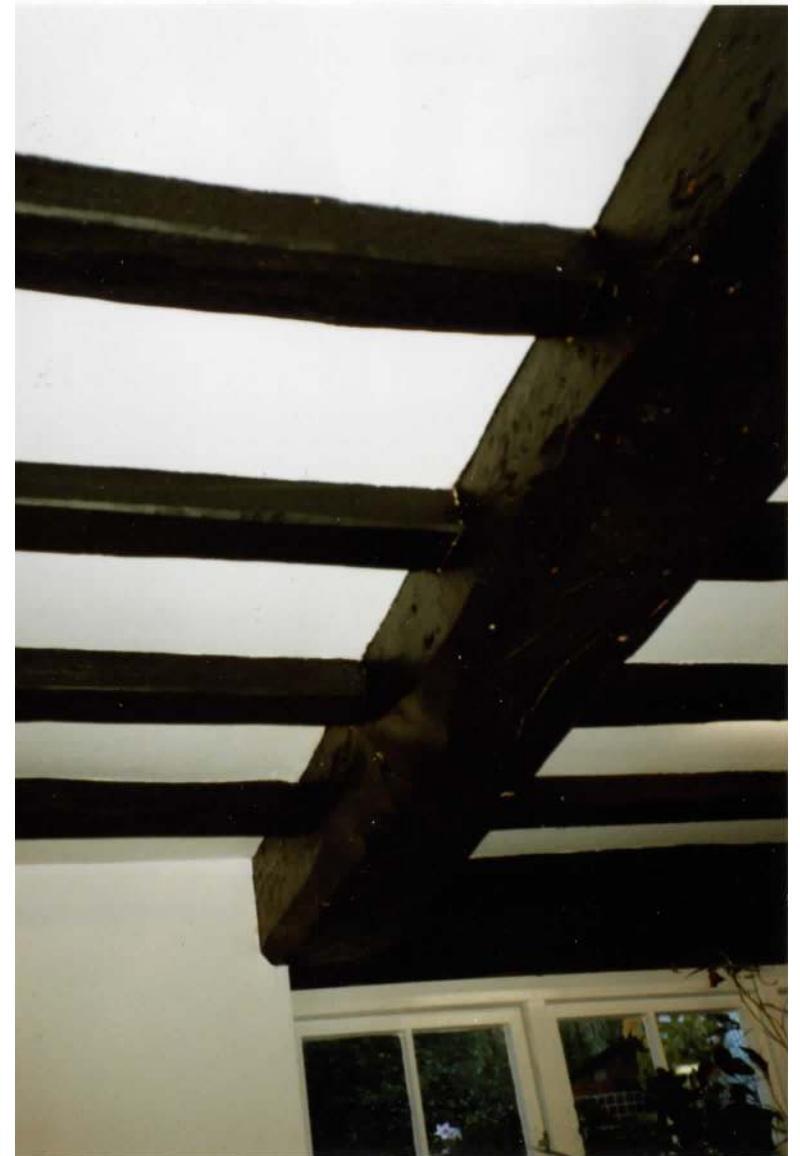
Kitchen Spine Beam, looking north
