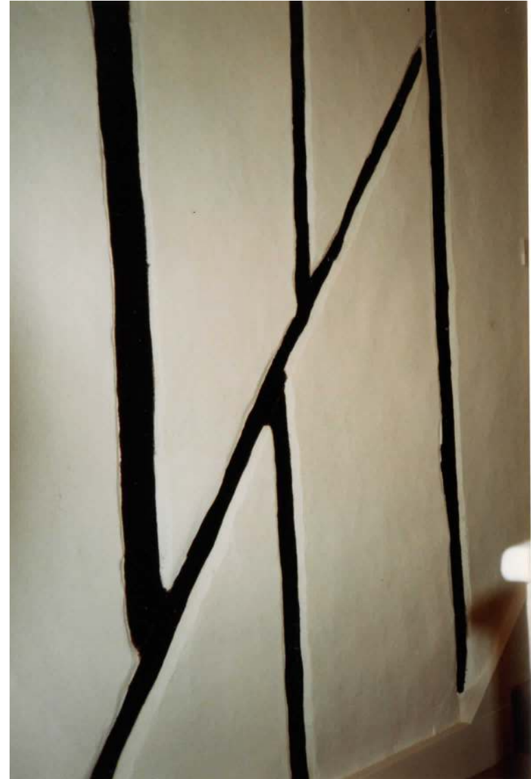
Studs in the East Wall of the Upstairs Rear Extension of No. 19 (denoting the former Roofline of the Cat's Slide Roof.)
