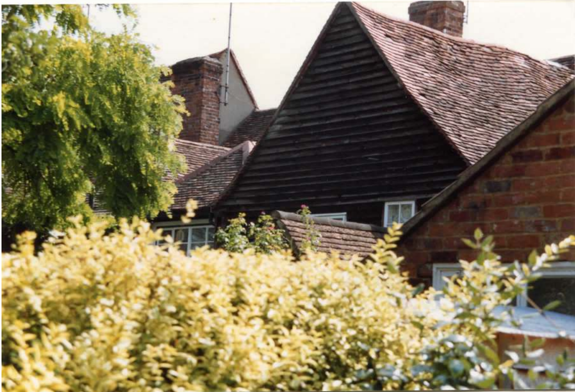
Rear Wing of No. 17 with Weather Boarded Gable. Low Kitchen Extension of No. 19 to the Left.
