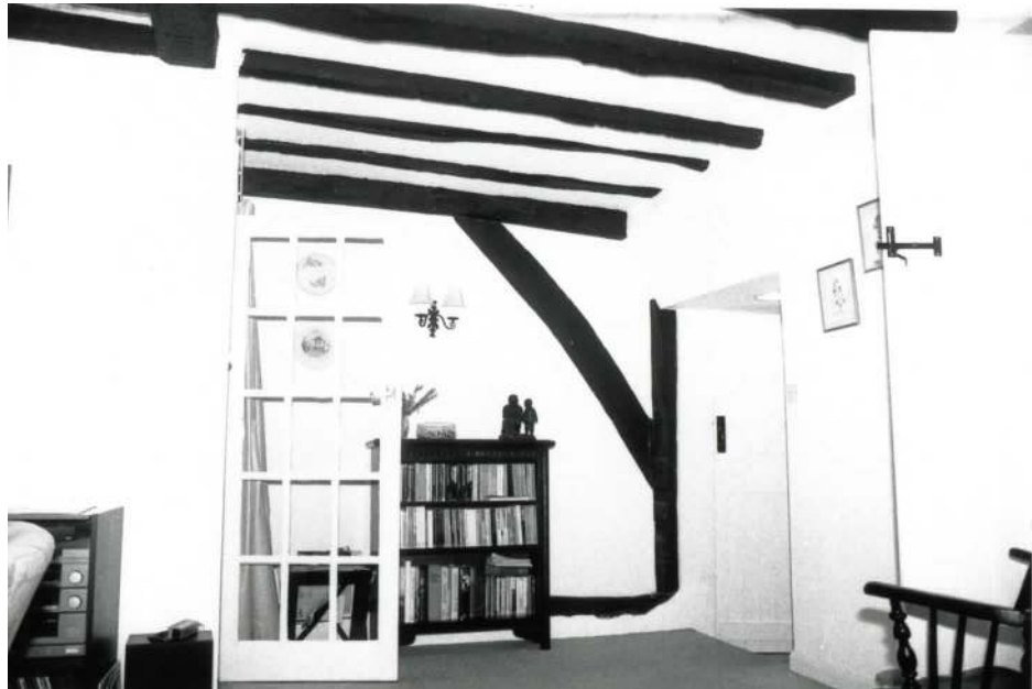
No. 17 Friday Street View from bay 2 into bay 1
