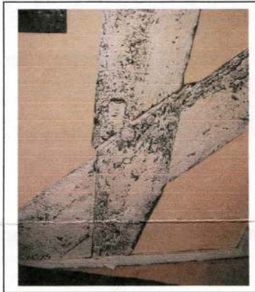
Front chamber with trefoil cusped window set into the close-studded frame of the east wall. NB the tension brace in the north/front wall; this is lap-jointed and pegged across the stud in the front wall.
