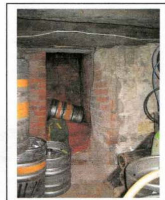
Above: NB recesses cut into underside of joists show the location of the former front wall. Right: Cellar – stone and brick & flint walls, heavy ceiling joists.
