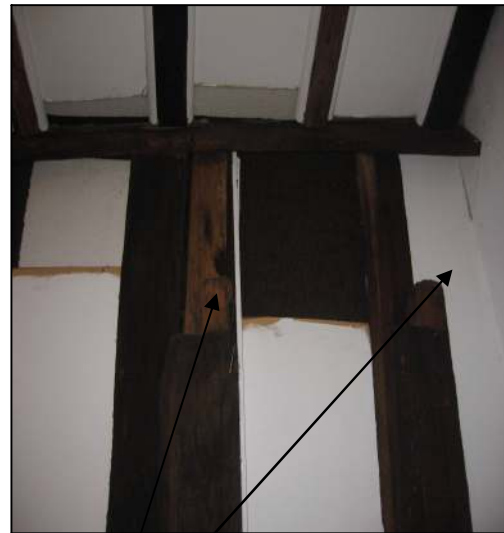
The two sooted, short rafters in bay II with their long tenons exposed. (NB these are not sooted as they would have been housed within the mortises of the louvre structure they once supported)
