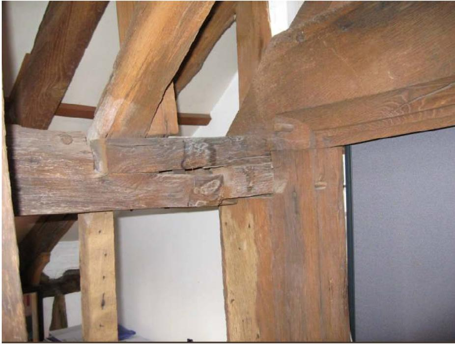
**Two sets of rafters visible in upper left of picture. The lower rafter rests on the wall plate putting strain on the ‘edge-halved, double bridled’ scarf joint creating a weakness in the structure.**
