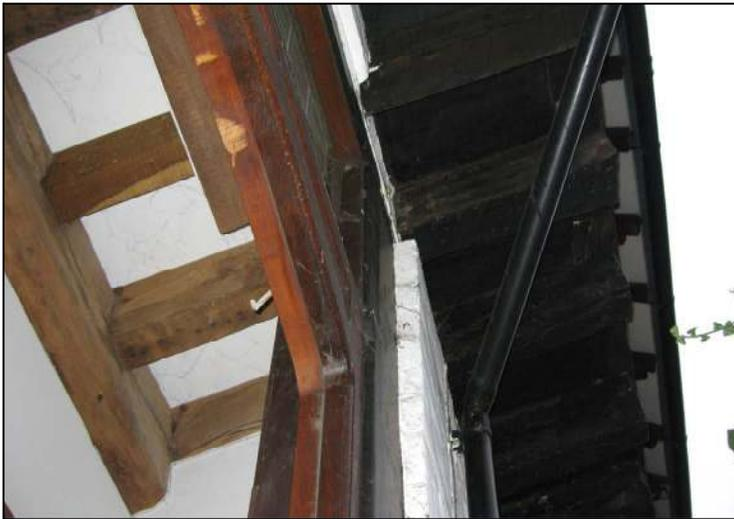
Short ceiling joists, tenoned into the restrainer beam on the left hand side and supported by the 2" Tudor brick wall in the middle (with modern door frame below), thus creating the jetty for the external gallery above, which would have been used as a link between the lodging ranges.
