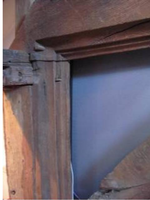
Hollow chamfer moulding in eastern post and tie beam, pt. of long arch brace just visible
