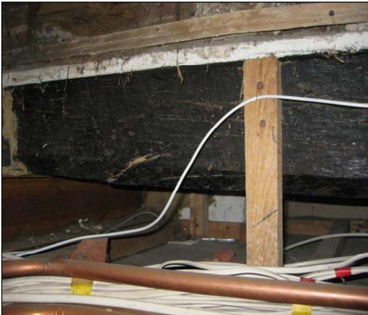
Back of the restrainer beam into which jetty joists are tenoned and which supports the timber stud wall above. This has been dendro dated to 1530.
