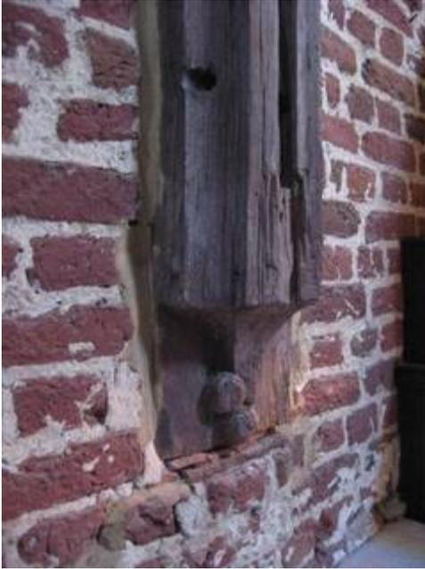
Carved balls as a pendant of the corbelled post, where it is set into the western brick wall. Empty brace slot above.
