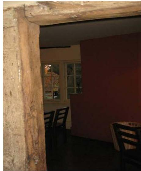
**Chamfered, mitred door opening in stud wall in the east range of the Old White Hart**
