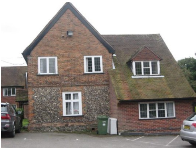
Highlands Farm House, b & f. parlour extension to timber framed house behind; with modern extension on the right. To be demolished to make way for modern 5-bedroom house and garage.
