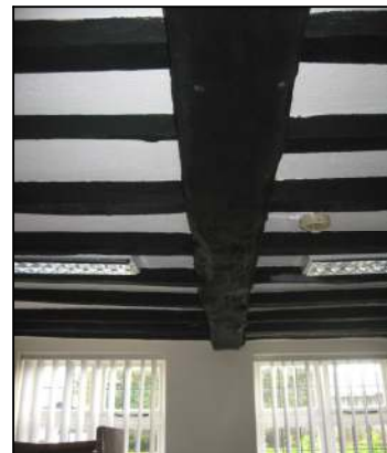
Left: Newel staircase seen from the attic; Centre: ceiling beams and coving for upper chamber fire place; Right: spine beam and ceiling joists. All above photographs are of the ‘new parlour wing’.
