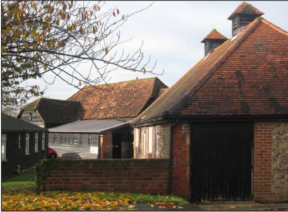
Barn and stable/cowshed group seen from the east gable of the stable, looking west towards the barn. The wide plank door in the gable suggests that the adjoining interior space once held the bull pen, ( a very similar bldg. exists at neighbouring Cowfields Farm) Note louvered ventilation turrets on the roof.
