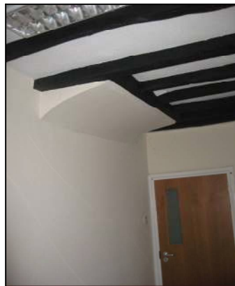
Left: Newel staircase seen from the attic; Centre: ceiling beams and coving for upper chamber fire place; Right: spine beam and ceiling joists. All above photographs are of the ‘new parlour wing’.
