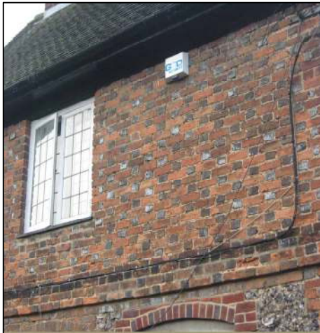
East front of C18 th brick work of tall, right hand building; a ‘Parlour Wing’ ? The central building has later brick walls encasing a two-bay timber framed structure. The dormers are modern, as are the roofs.
