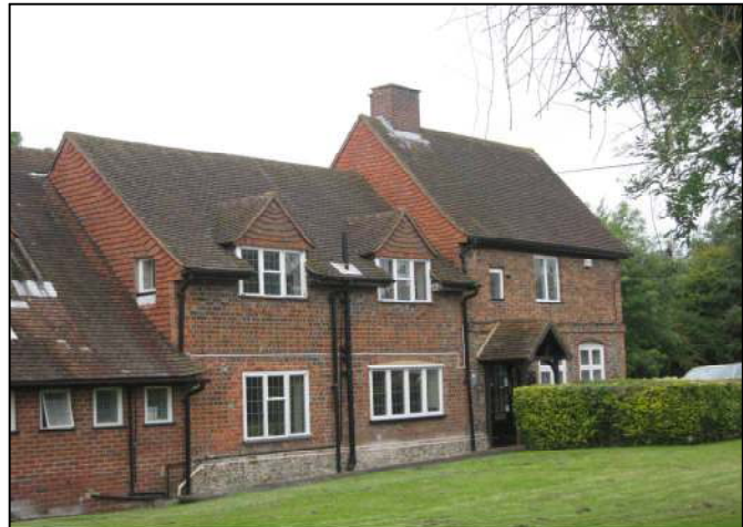
East front of C18 th brick work of tall, right hand building; a ‘Parlour Wing’ ? The central building has later brick walls encasing a two-bay timber framed structure. The dormers are modern, as are the roofs.
