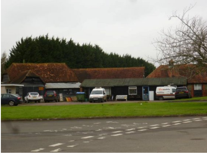
Existing Barn Group (behind modern sheds) protecting the north side of the farmyard. These barns are to be demolished under the proposed scheme and replaced with the above block of flats.
