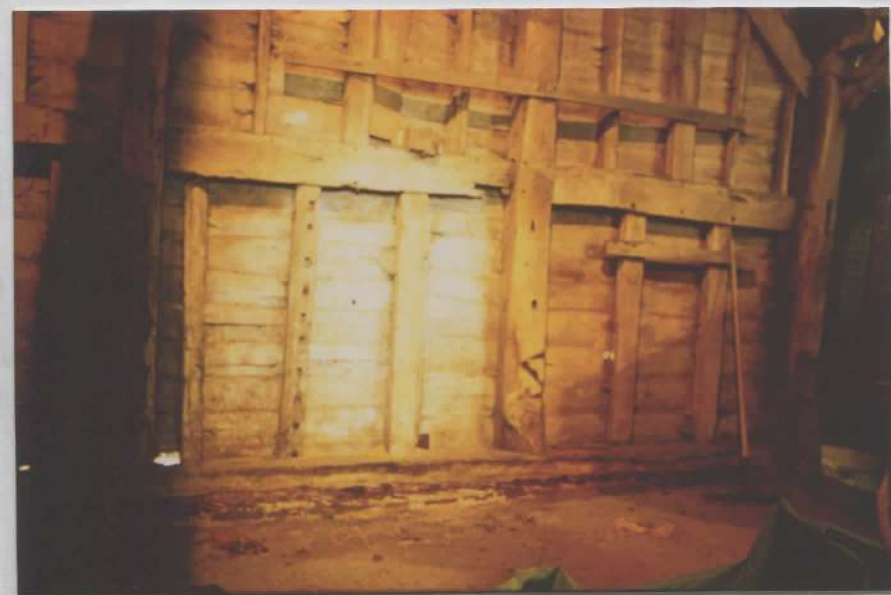
East side, bay 4 showing low plinth of tiles
