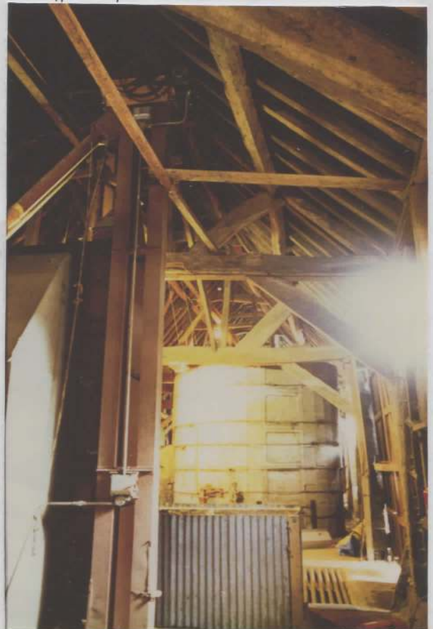
West side, bay 6 looking south
