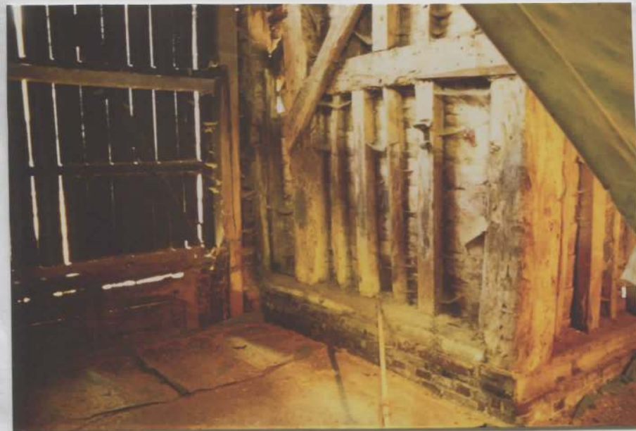
East side, porch in bay 6
