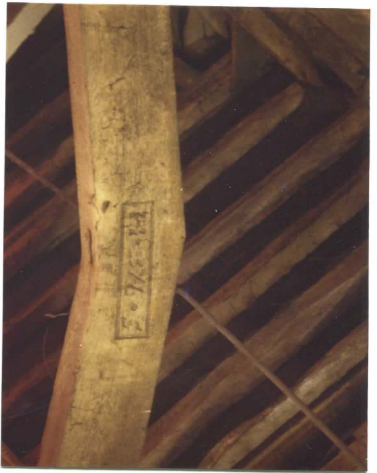
Collar of Truss D-D1
