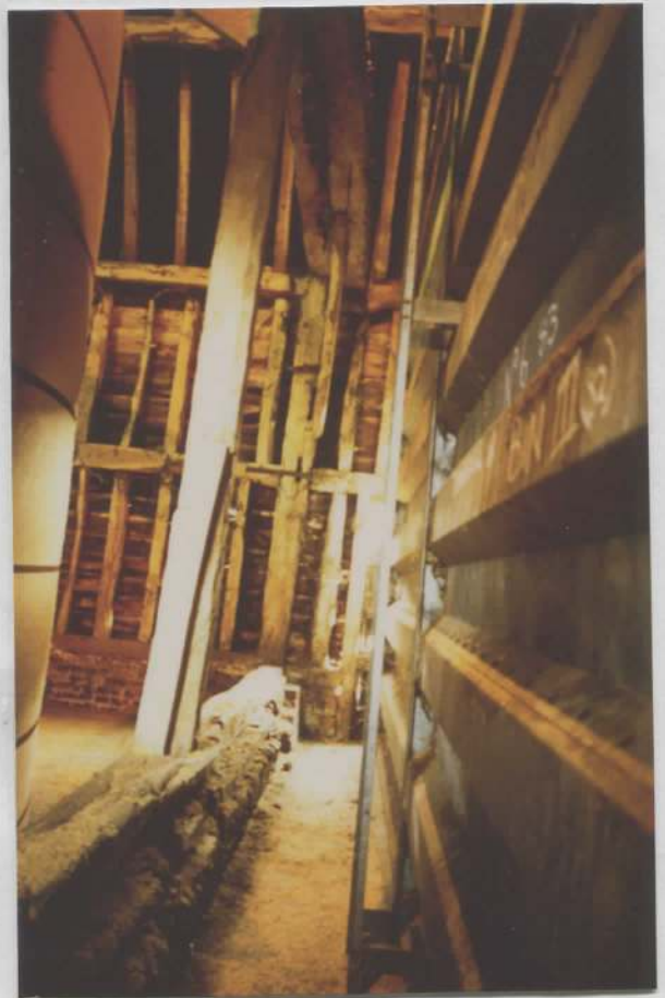
Truss B-B1 showing former outside wall with brick & flint off-set plinth.
