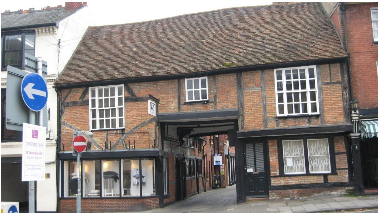
North front elevation of Nos 45 /47 Market Place, formerly the 'Broad Gates'
