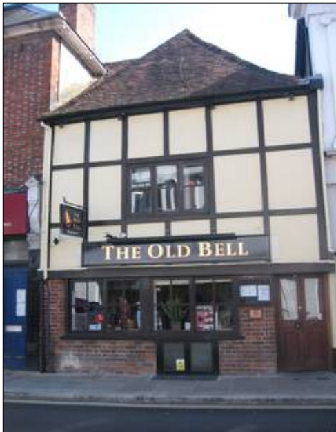
20 Bell Street, west/front elevation showing hipped roof, which replaces gable of 1325 date
