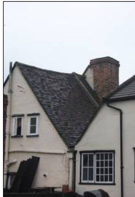
20 Bell Street, l.h.side, east/rear elevation. N B difference in roof heights
