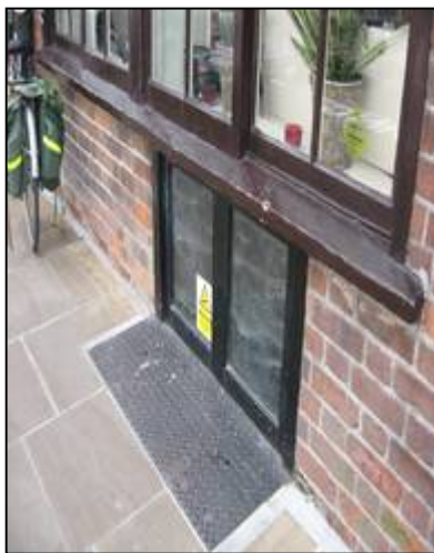
Cellar access from the street
