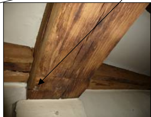
Below: Spine beam with chamfers and stops in Bay II
