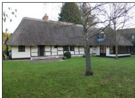
West rear elevation, square panel framing
