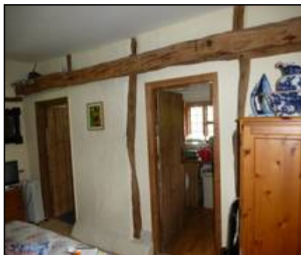
North wall of Bay III
