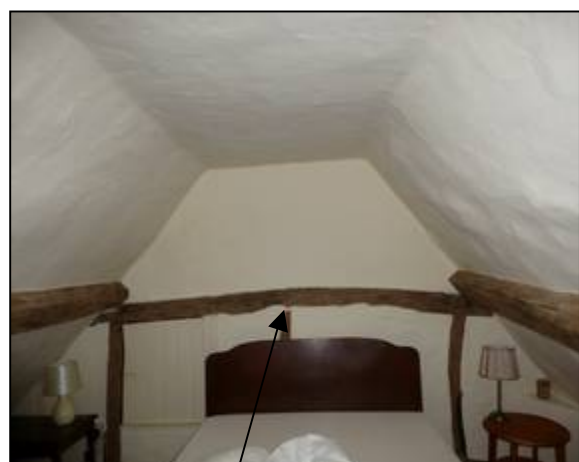
Clasped purlins and the three queen struts between tie beams (not visible here) and collars
