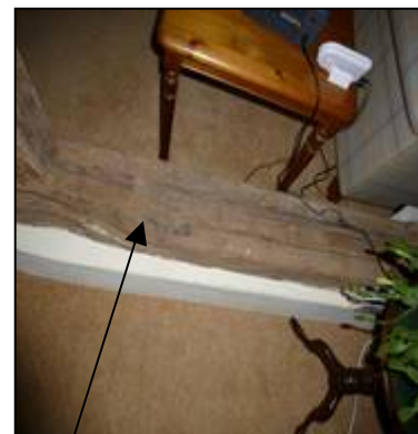
Above: Sill beam with groove between Bays I and II
