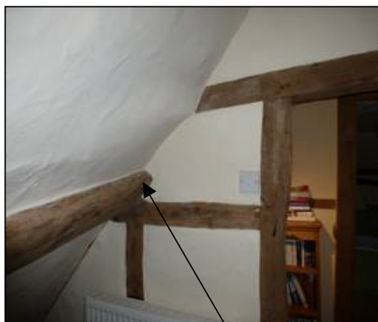
Clasped purlins and the three queen struts between tie beams (not visible here) and collars
