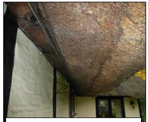
1 m thick thatch at rear/west wall
