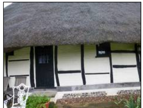
External view, west wall of Bay III
