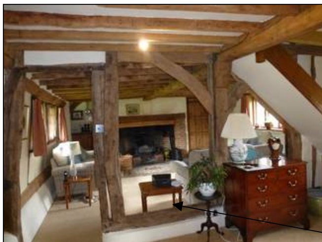
Above: Sill beam with groove between Bays I and II
