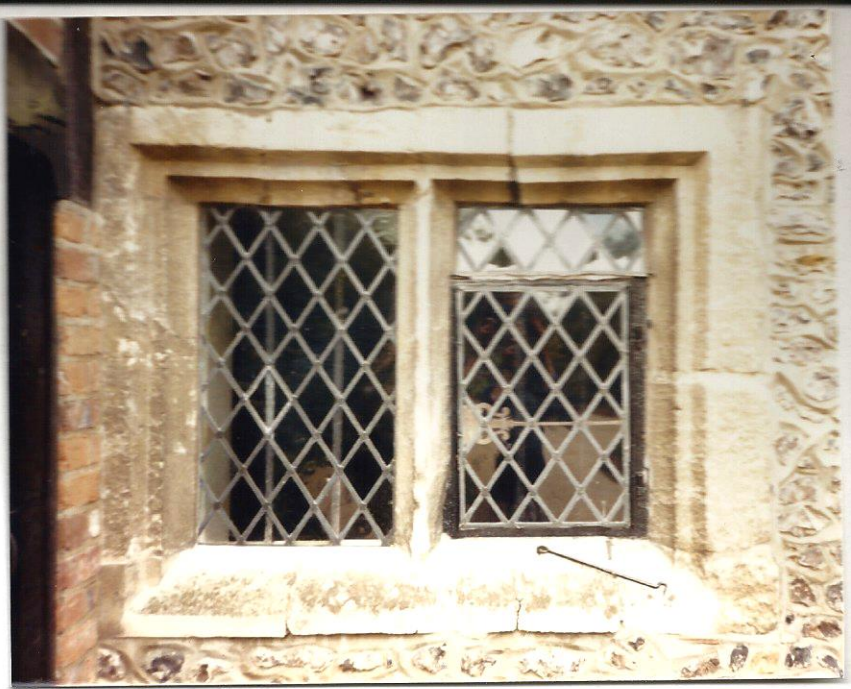
Original window with stone mullion & iron casement Front door
