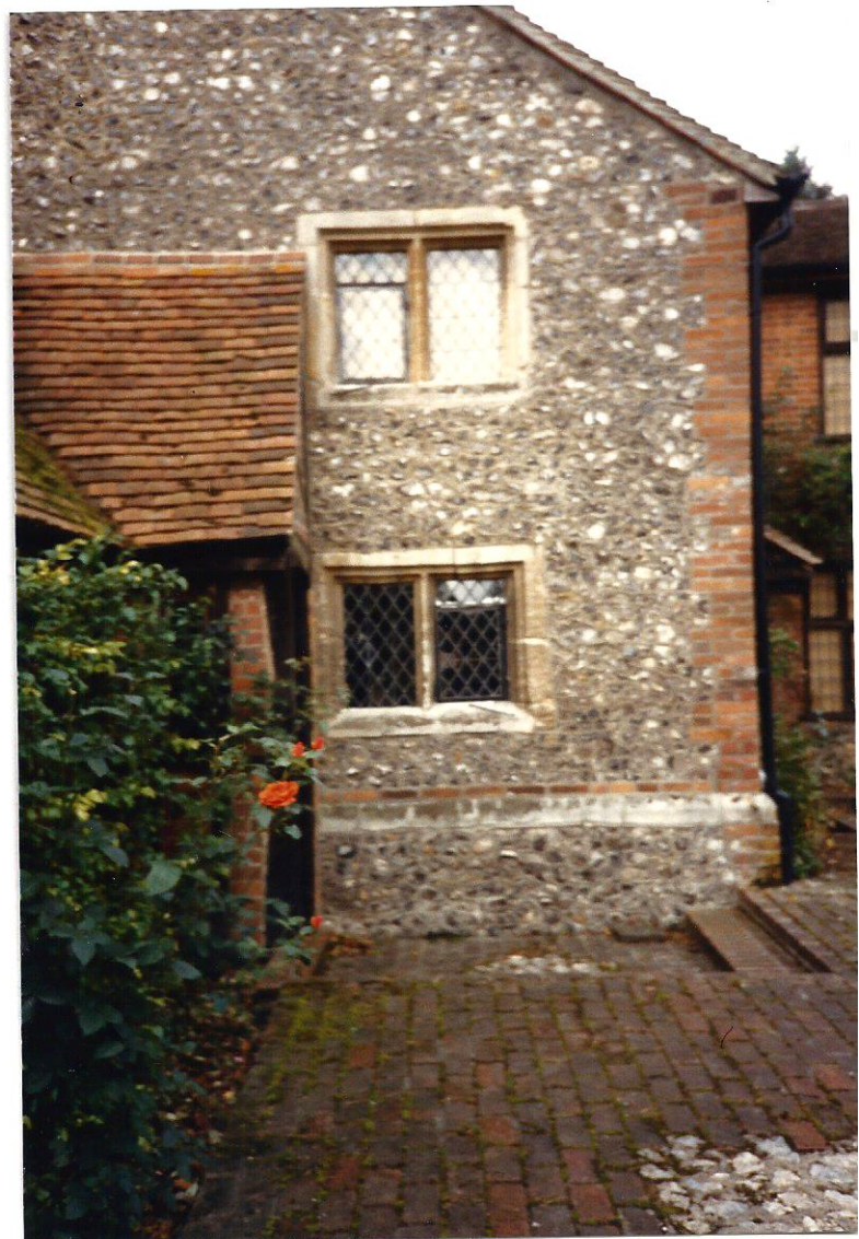
back outshut with orig. windows (see close-up above)
