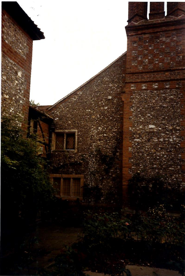
Westgable outshut, modern extension to the left
