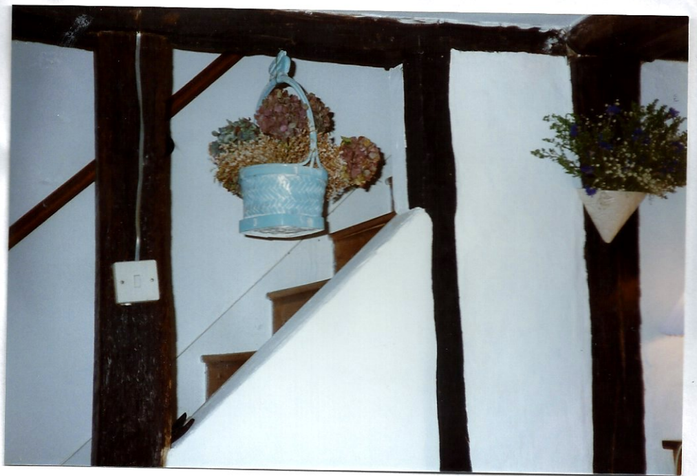
Partition wall and staircase
