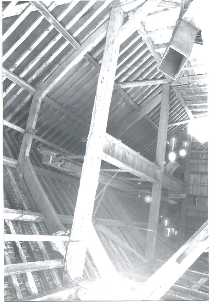
Barn IV with cob wall
