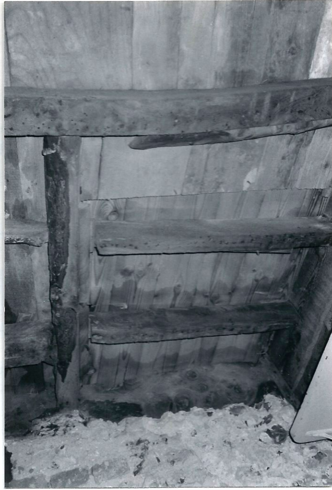
BAY II, ceiling timbers, pos-former access to 1st floor.
