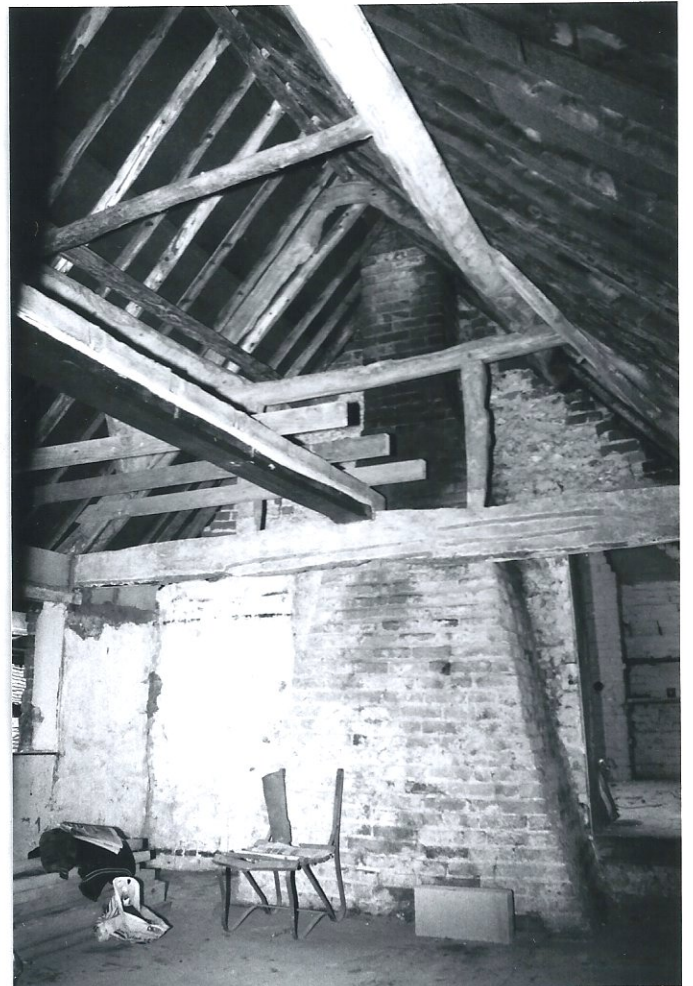
'FLINTS' BAY I, repointed chimney stack 1st floor BAY I stack and now demolished ex- tension
