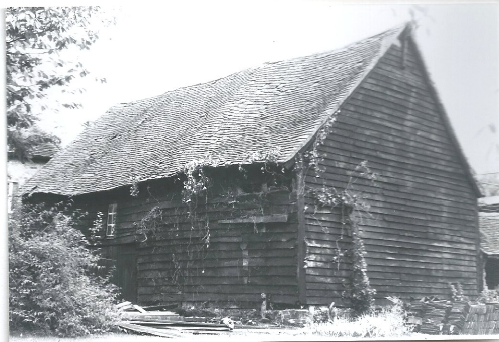
South gable and west side of barn.
