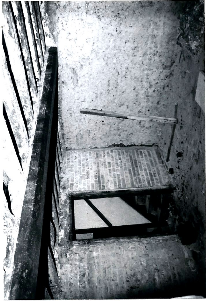
BAY I, access to outdoors and stairs
