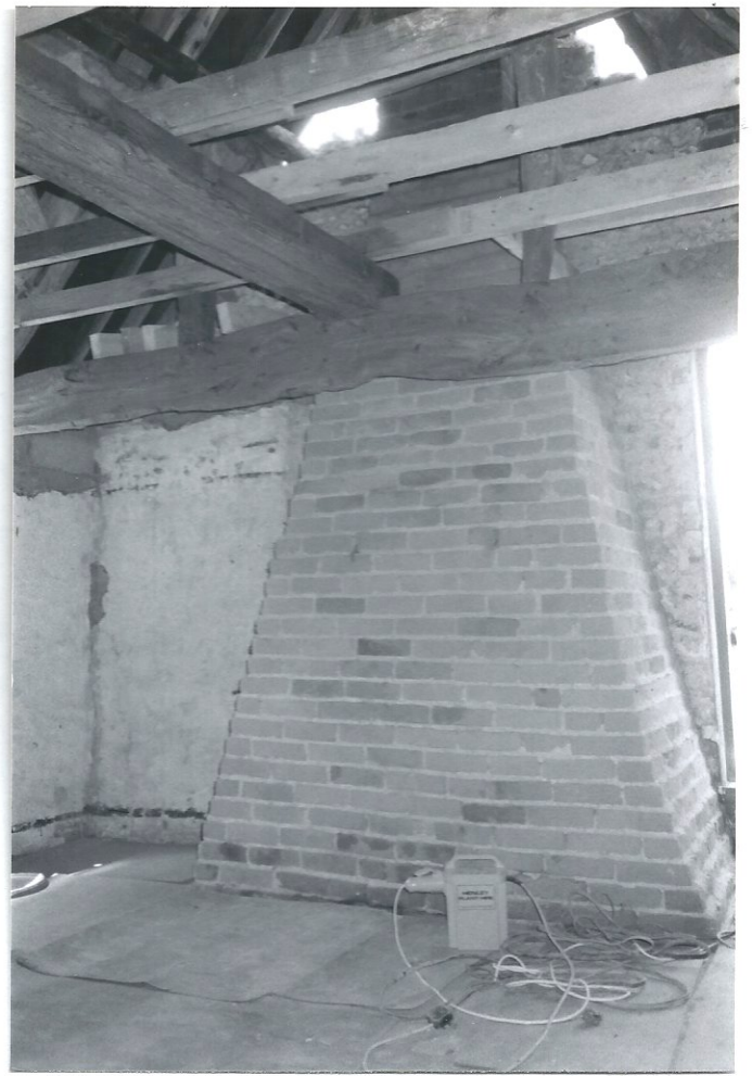
'FLINTS' BAY I, repointed chimney stack 1st floor BAY I stack and now demolished ex- tension
