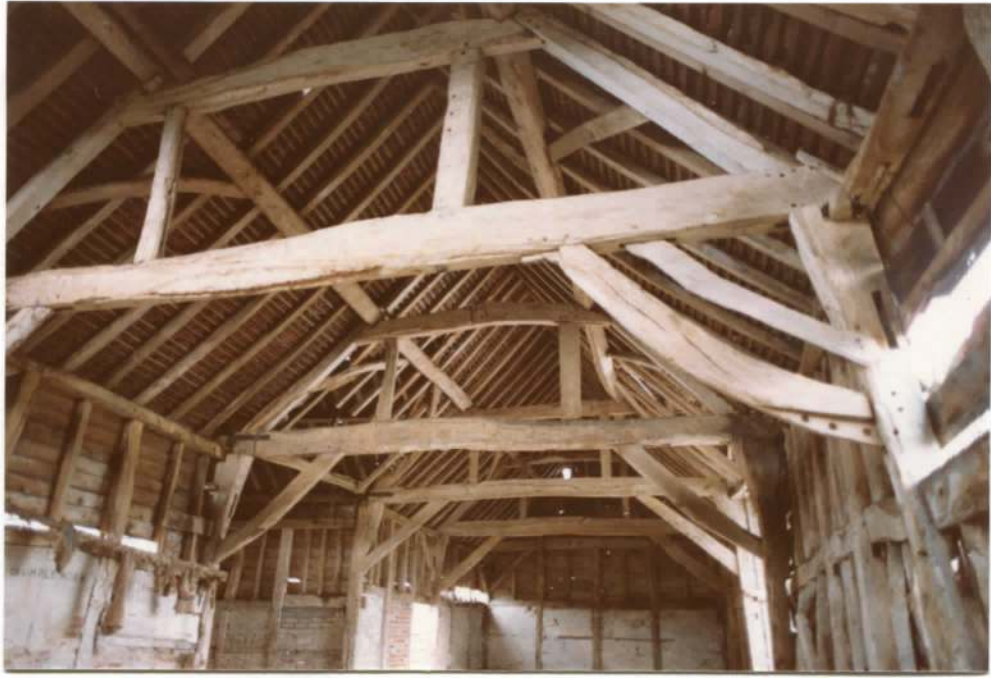
Barn before conversion, note brace post on right (re-used)
