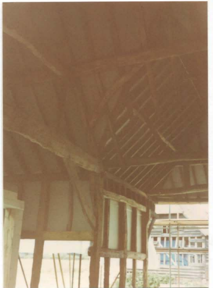
During conversion; porch. 1983 R. Gisson
