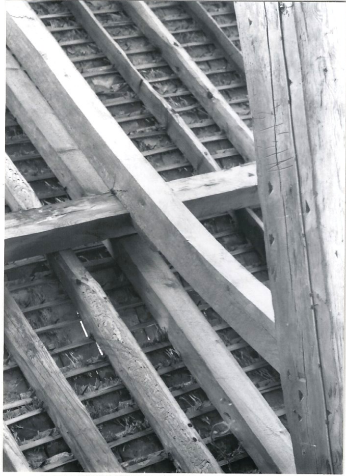
Tie beam & inner curved principal rafter supporting purlin
