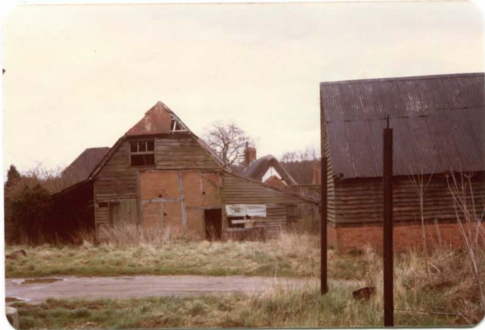
Binfield Heath Bournes Farm, Barn, North-West gable, looking towards 'Bottle & Glass' P.H.
