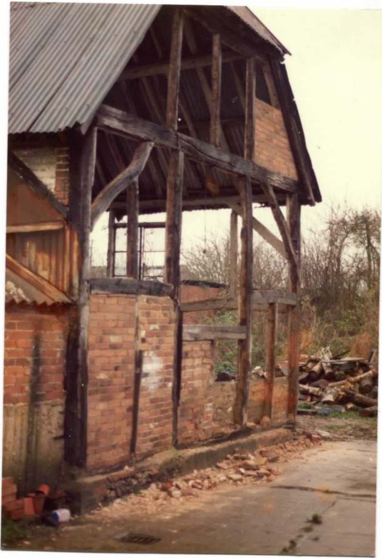
Bournes Farm Barn c.1983/84
