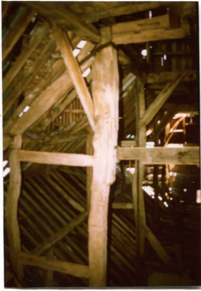
Truss C, looking west
