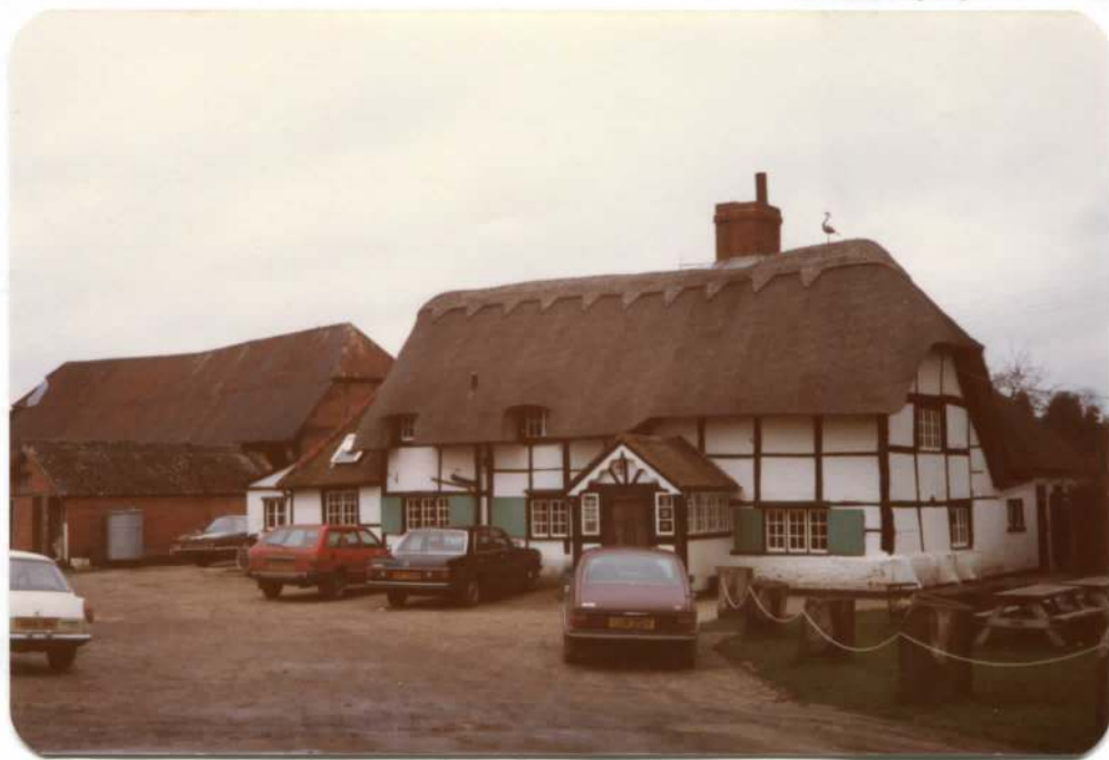
Looking at the barn from 'Bottle & Glass' P.H. which is very probably the original Bournes farm house.
