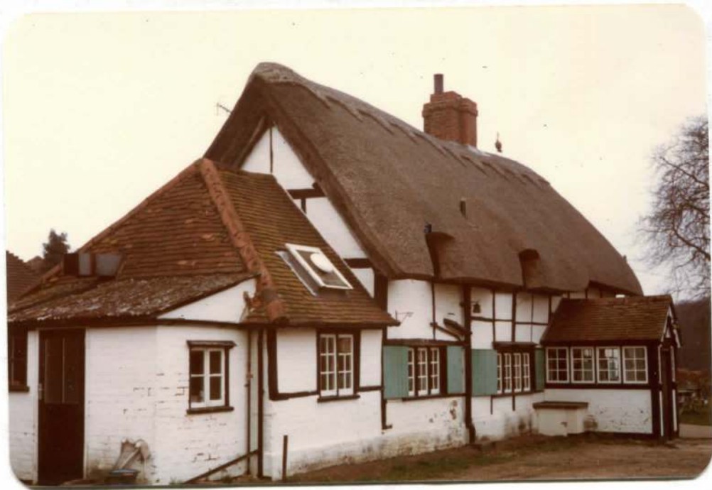
North-West Gable with extensions
