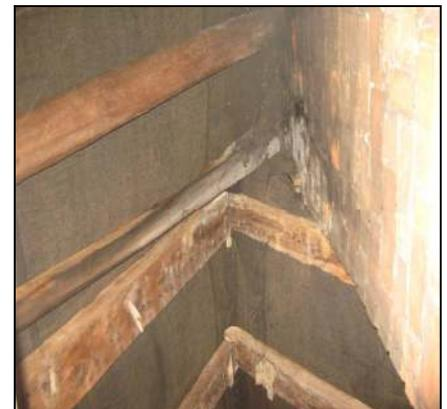
View of the rafters from the attic lobby behind the central brick stack. The rafters are apex pegged
