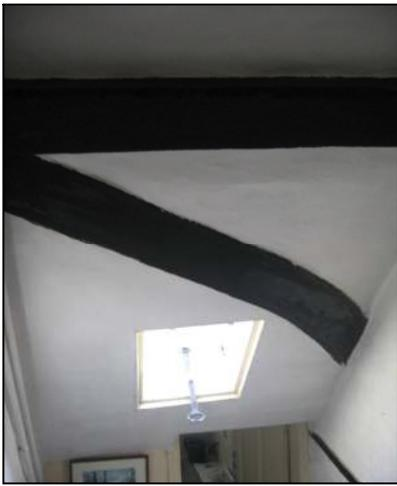
The upper floors are reached by a 19<sup>th</sup> C stair case from the rear lobby. Although modernized, extended and altered the main body of the stairs still occupies its original space to the rear of the stack. The wind braces of the attic roof, under which it rises, are visible on its south side (photograph on the left)
