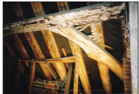
Right: roof with cusped wind brace
