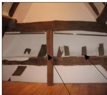
Sooted central truss at No. 9 No. 11. Left: Open western crown strut truss; rafter feet and purlin of No. 13 beyond NB. New rafter inserted above Right: Eastern closed truss with wide, cambered collar; w & d infill. Does it increase the roof height? NB. Trusses were sooted before recent modernization
