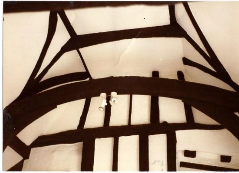
Cambered tie beam & braces looking west - on plan -
