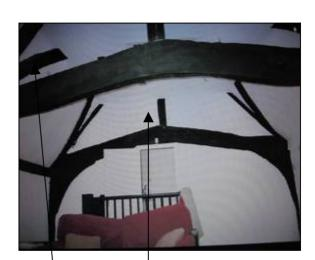
L. h. picture: Part of the east gable with fire place of the 'Barn' (Truss A and Truss B in the foreground). Note the central post which rises to the tie beam. Above it another central strut rises to the collar, also known as a crown strut. All other narrower studs are part of the wall infill, which support the wattle and daub panels.
