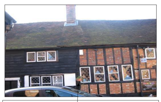
The continuous roof and single wall post (Truss A on plan) show that the weather boarded and the timber and brick sections are very likely of one build. Neither external walling materials are original; this would very likely have been wattle and daub making up the panels between wall posts, studs and rails.
