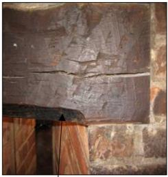
Fireplace inserted below eastern truss. This is part of a 2-flue stack, which also serves the first floor flat (Bay V d). The central brick hearth is a 20<sup>th</sup> C. addition. On the left is the former access, now blocked, to the south lodging range, now the g.f. entrance to the flat.
