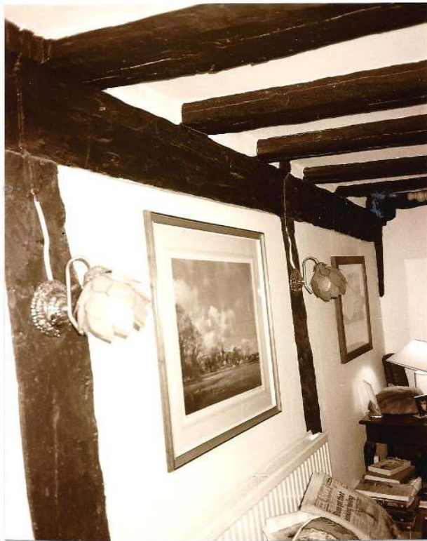
BAY II, ground floor, showing large wall panels, low sill and wide ceiling joists
