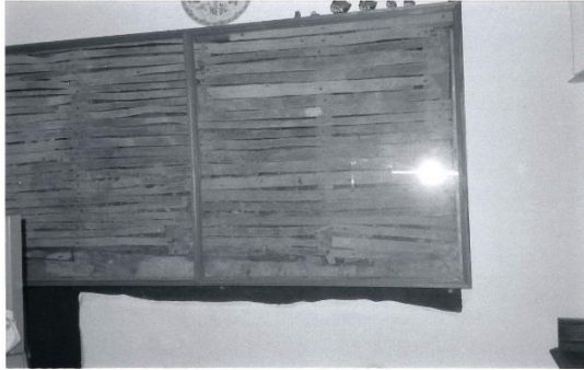
1st floor, west wall, lath & plaster panels
