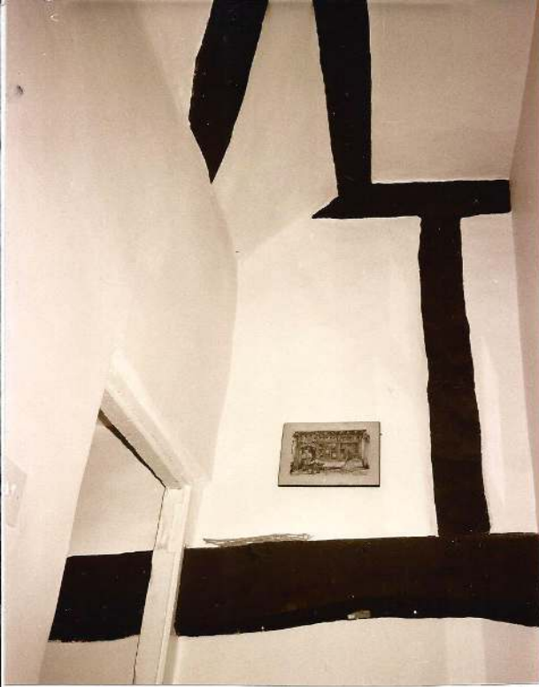
Truss in west gable, BAY II showing cambered tie, queen's posts & curved windbrace
