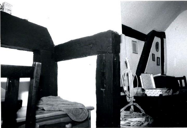
Cut through south wall, BAY 1st floor
