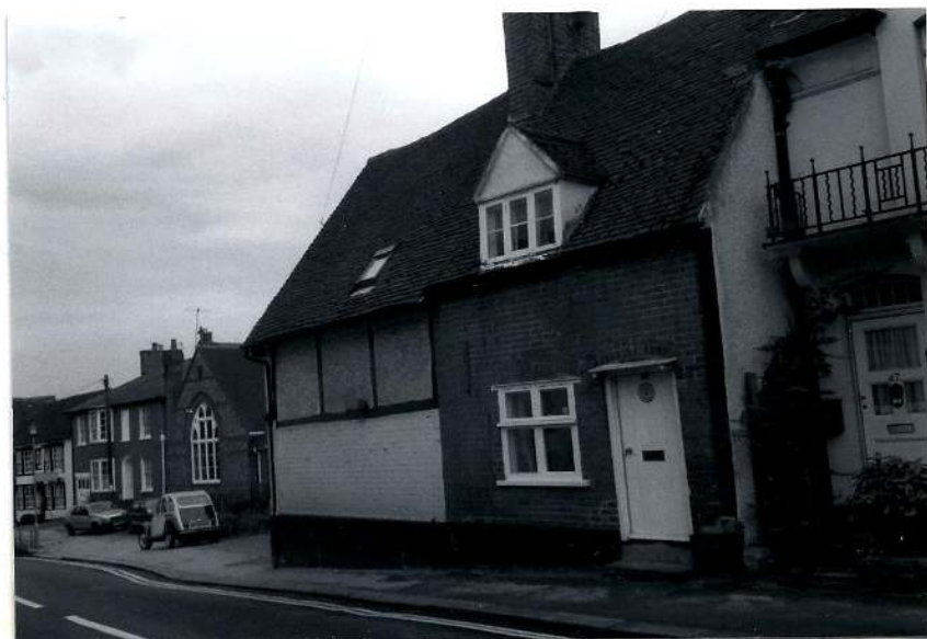
North front Nos. 43 & 45 Gravel Hill.
