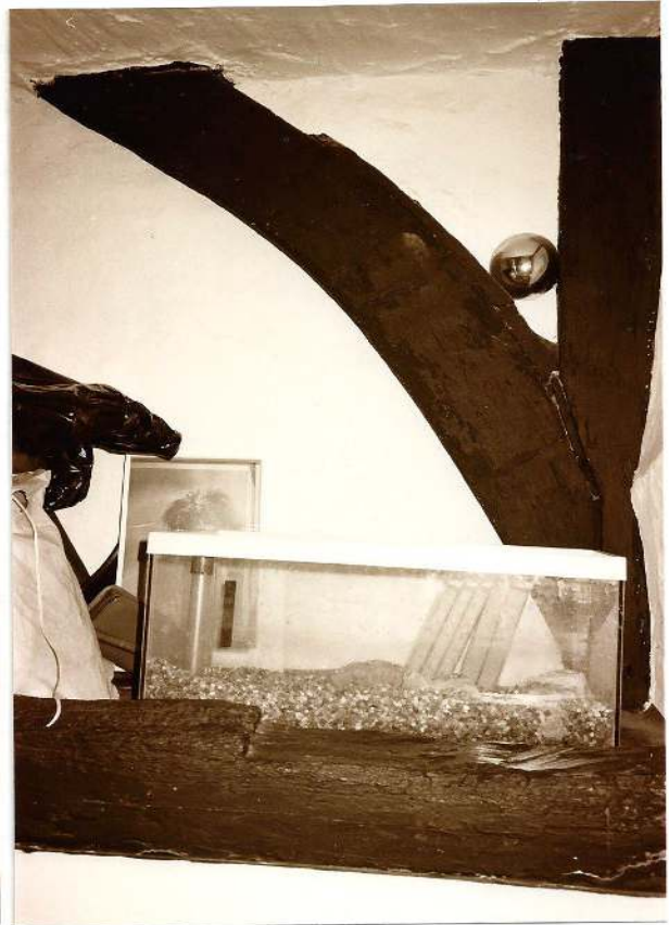
Studwall, BAY II, note former dooropening Central Truss with Girthing Joist at 1m distance in front
