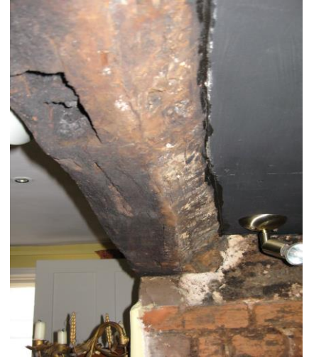
Ingenook with timber bressumer with deep, sooted chamfer in western front room.
