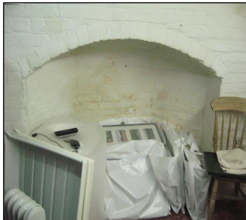
Brick stack relieving arch in the cellar
