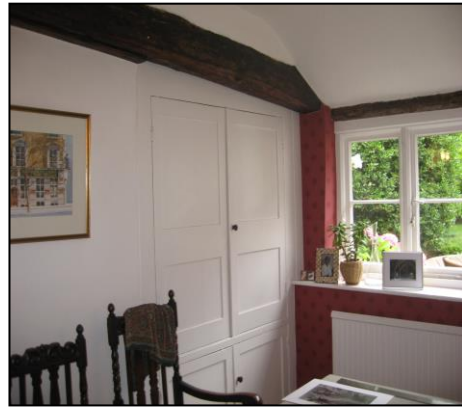
East wall with exposed, straight cut plate; below are the doors to the external cupboard.
