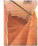
Newel stair in rear stair turret 023
