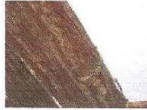
Lambs tongue stop in ceiling beam 015
