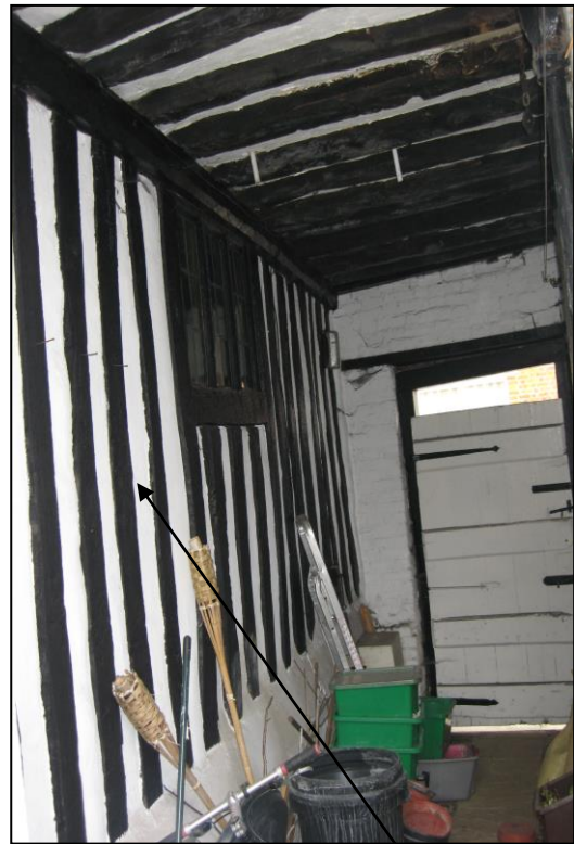
Interior of passageway with the close studded timber frame and early C17 th mullion window of No 14 on the left
