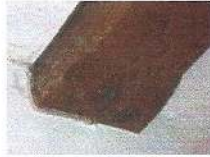
East front room ceiling beam stopped 008
