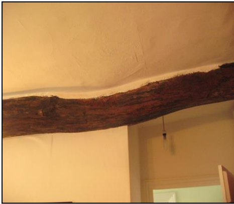
Very curvy west wall plate indicating lack of good quality timbers
