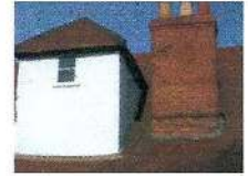
Stair turret and main stack 4.3.10 003
