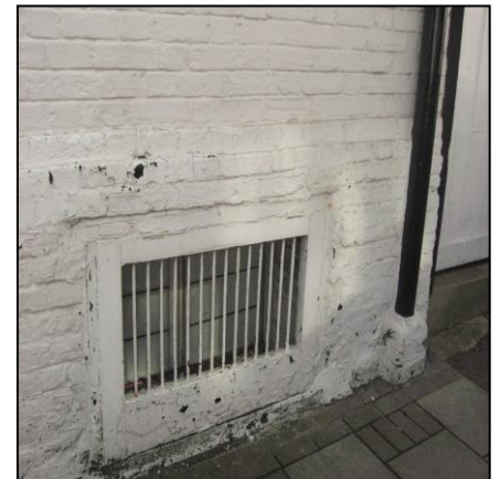
Barred delivery cellar opening
