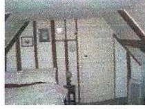
Attic cross wall 021
